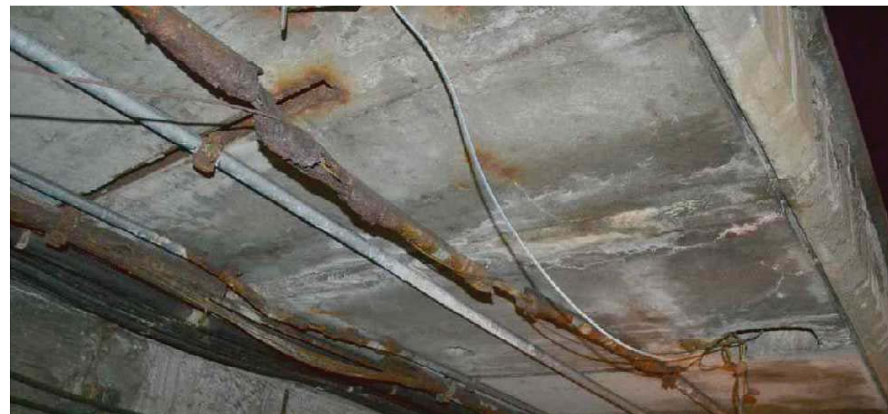
CORRODED CONDUIT DETAIL: PHOTO A A11E-100 SCALE: NOT TO SCALE
