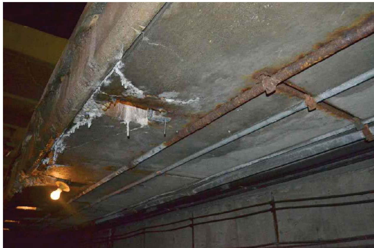
CORRODED CONDUIT DETAIL: PHOTO A A11E-100 SCALE: NOT TO SCALE
